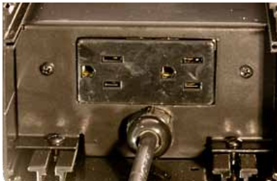
Bottom view - Dual Grounded Receptacles
